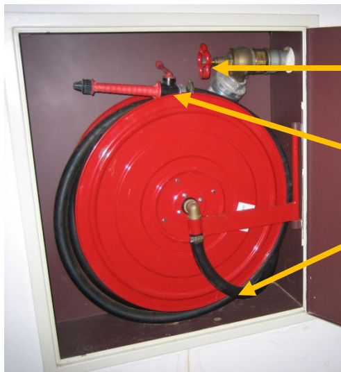
pic.4.4.2: opened wall hydrant cabinet
