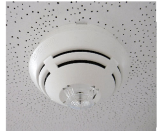
pic. 4.2: smoke detector
