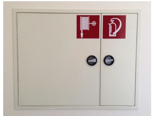
pic. 4.4.1: wall hydrant cabinet (here together with extinguisher)
