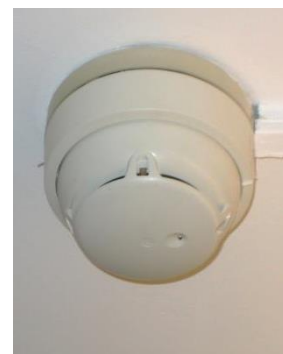
pic. 4.2: smoke detector
