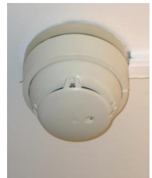
pic. 4.2: smoke detector
