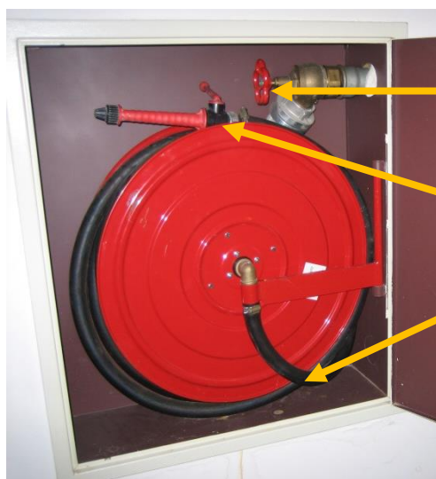
pic.4.4.2: opened wall hydrant cabinet
