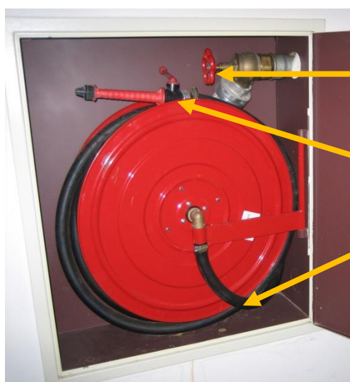
pic.4.4.2: opened wall hydrant cabinet
