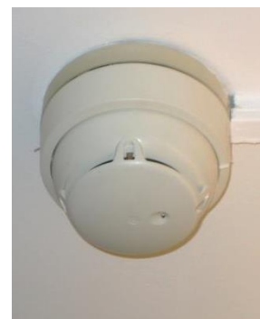
pic. 4.2: smoke detector
