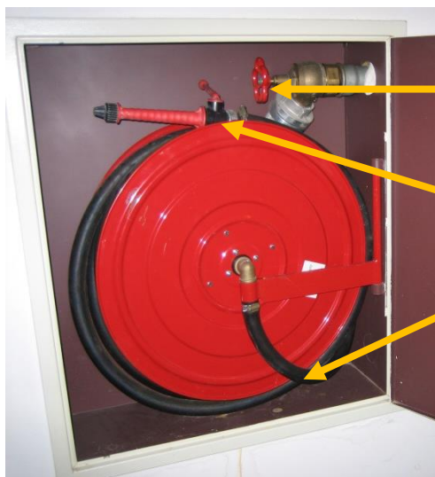
pic.4.4.2: opened wall hydrant cabinet
