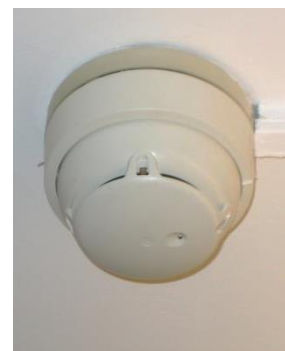
pic. 4.2: smoke detector
