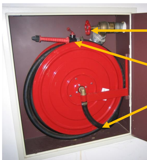
pic.4.4.2: opened wall hydrant cabinet
