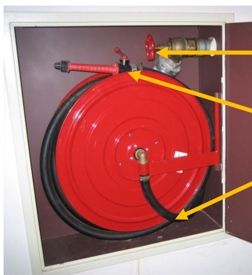
pic.4.4.2: opened wall hydrant cabinet
