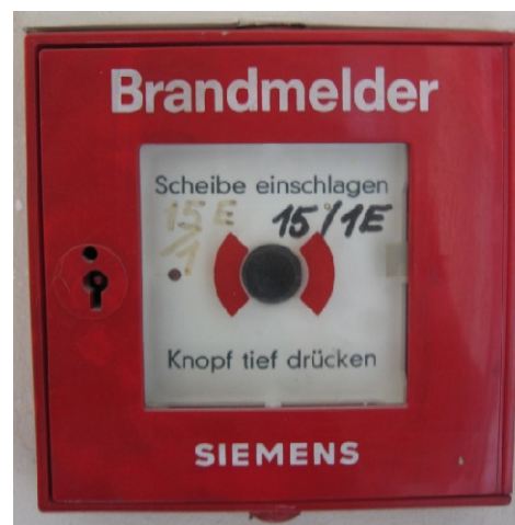
Pict. 1: Fire Alarm Button
