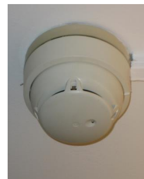
Pict. 2: Automatic Smoke Detector
