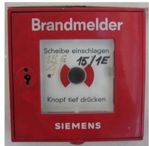
Pict. 1: Fire Alarm Button
