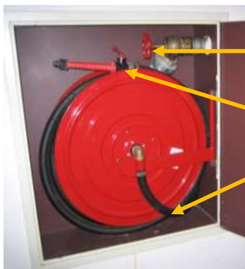
pic.4.4.2: opened wall hydrant cabinet
