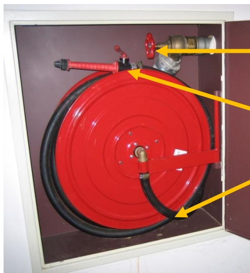
pic.4.4.2: opened wall hydrant cabinet
